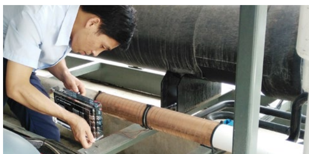
Installation de Vulcan S100
