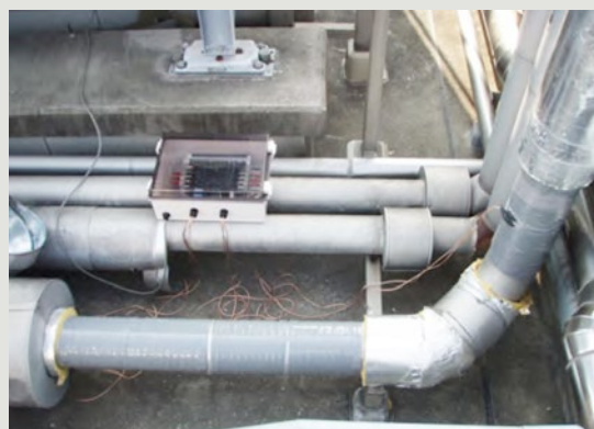
Installation de Vulcan S100
